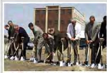
Stephen Goldsmith and Jessica Nava of Artspace break ground for the Bridge Projects with donors and members of Artspace's Board of Trustees.
